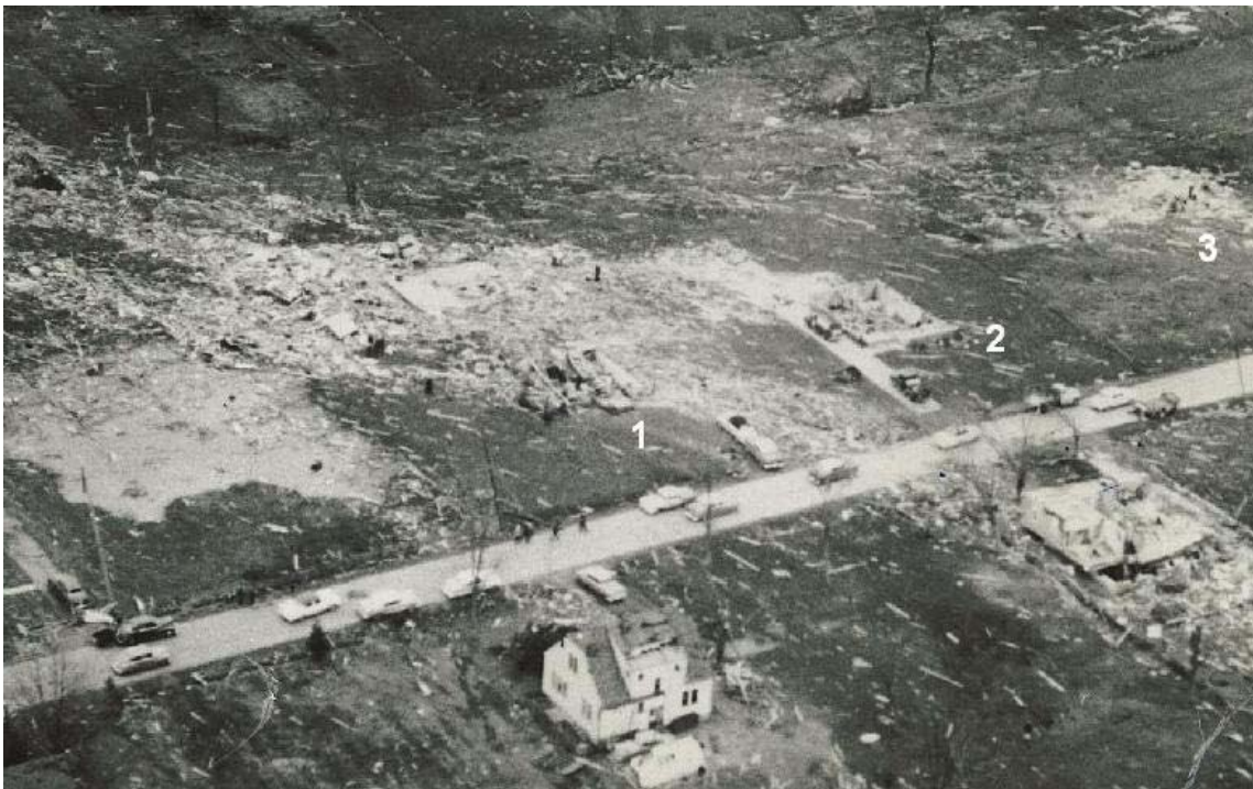
Figure 15: (a) Aerial photo of damage on New Holland Street in Hudsonville, MI. Four empty foundations mark the locations of homes that were swept away. The foundation of the Willard Brower home is labeled 2. Photo credit: Pete Ludema. (b) The Willard Brower home in 1954. Photo courtesy of Maxine Baker. (c) The foundation of the Willard Brower home. Photo courtesy of the Gary Byker Library.
