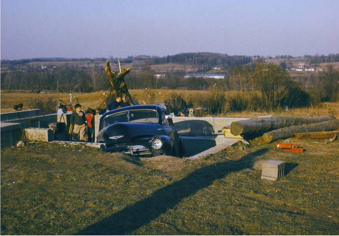
Figure 11: A car sits in the foundation of a home near Rockford, MI, after being hit by the Hudsonville to Lakeview tornado. No injuries resulted as the house was vacant at the time. At least two other homes in this area were destroyed and several others had extensive damage. There is no indication how or if this home was secured to its foundation, therefore winds in the F4 range cannot be inferred. Photo credit: Jack Erickson.
