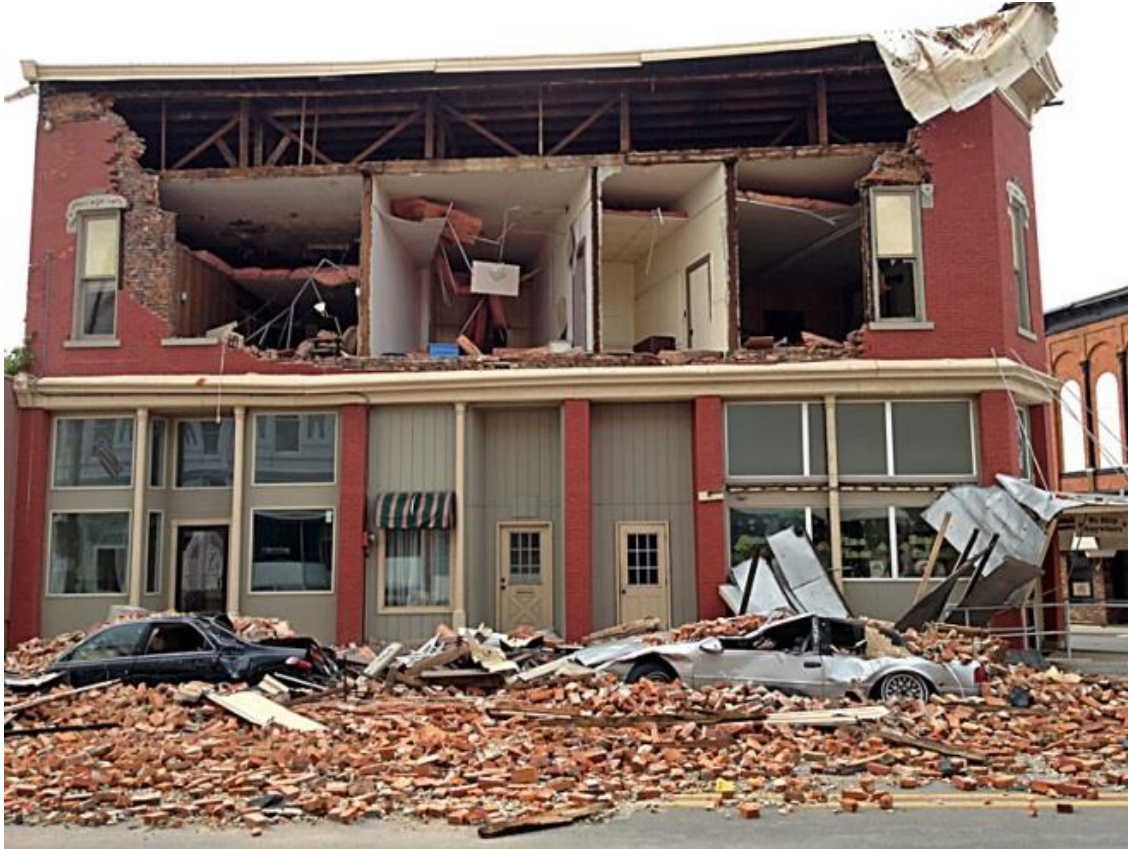
Figure 13: Bricks lying on top of two cars after a second-story brick wall collapsed from a storefront in Columbus Grove, OH. [Photo credit: Eric Davis.]
