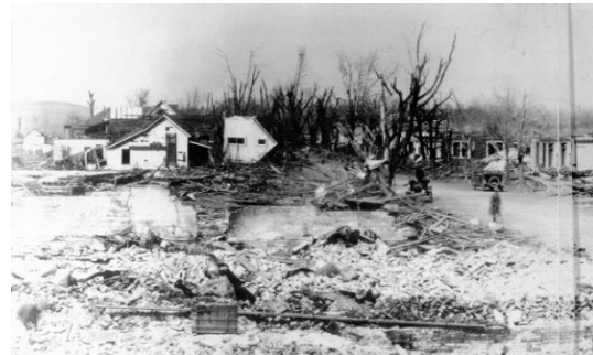
Figure C8: Photo from central Griffin, looking north. In the foreground are destroyed homes, with only partially or slightly damaged homes farther north. Not seen in the photo is another area, even farther north, with destroyed homes. This and other photos, and other evidence mentioned in this section, support the concept of a multi-vortex tornado passing through Griffin and producing significant damage gradients. Photo courtesy of the New Harmony Library, Posey County, IL.
