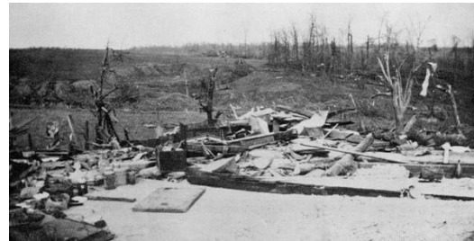
Figure C3: The destroyed home of Judge Claus Stueve. Photo courtesy of Carla Jordan, Lutheran Heritage Center & Museum of Altenburg, MO.
